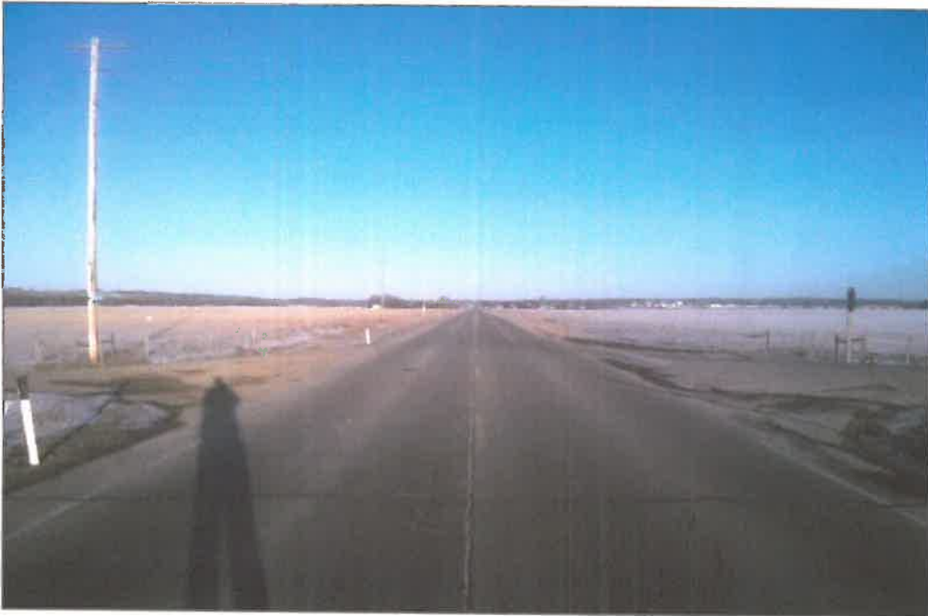
Photo 2: Intersection of Highway 584/Range Road 61 – looking east on Highway 584
