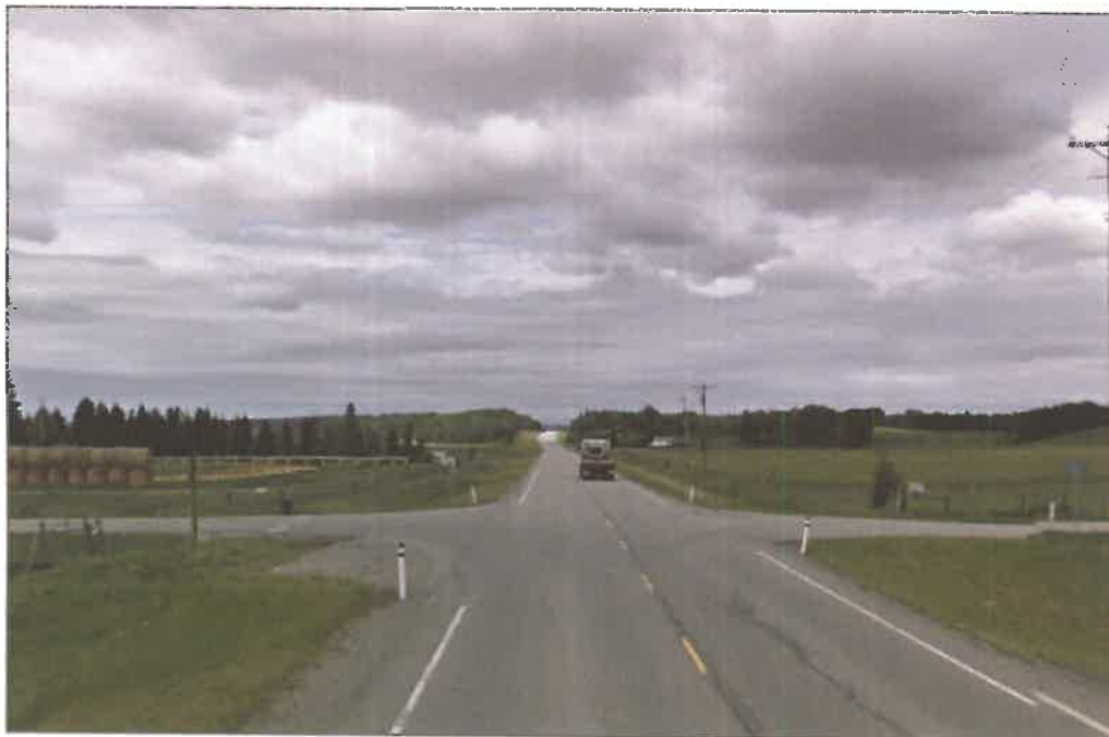
Photo 6: Intersection of Highway 584/Range Road 61 – looking west
