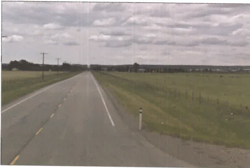
Photo 8: Highway 584 – looking east from Range Road 61
