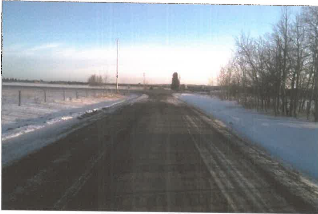
Photo 7: North leg of Range Road 61– looking south towards Highway 584
